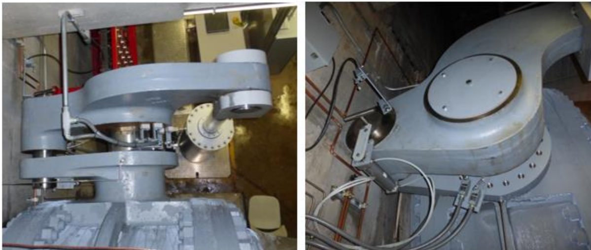
Figure 19–19. Top view (left) and side view (right) of a pneumatically actuated locking pin with manual handle in a horizontal valve's hydraulic operator's exposed linkage
