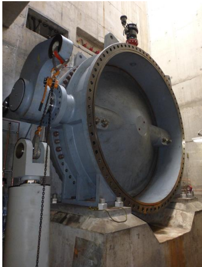
Figure 19–2. Flanged horizontal butterfly valve with hydraulic operator and lenticular disk (shown unlinked) with scroll case extension removed
