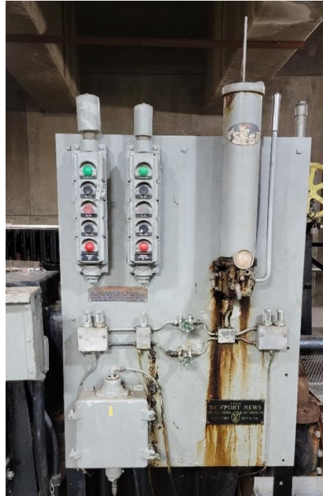
Figure 19–25. Valve grease pump and distribution manifolds (metering valves) leaking
