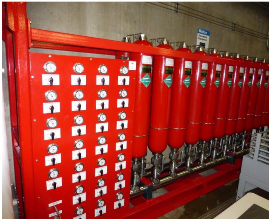
Figure 19–20. Valve operator hydraulic accumulator bank with individual take isolation valves (bottom) and pressure gauge panel (right)
