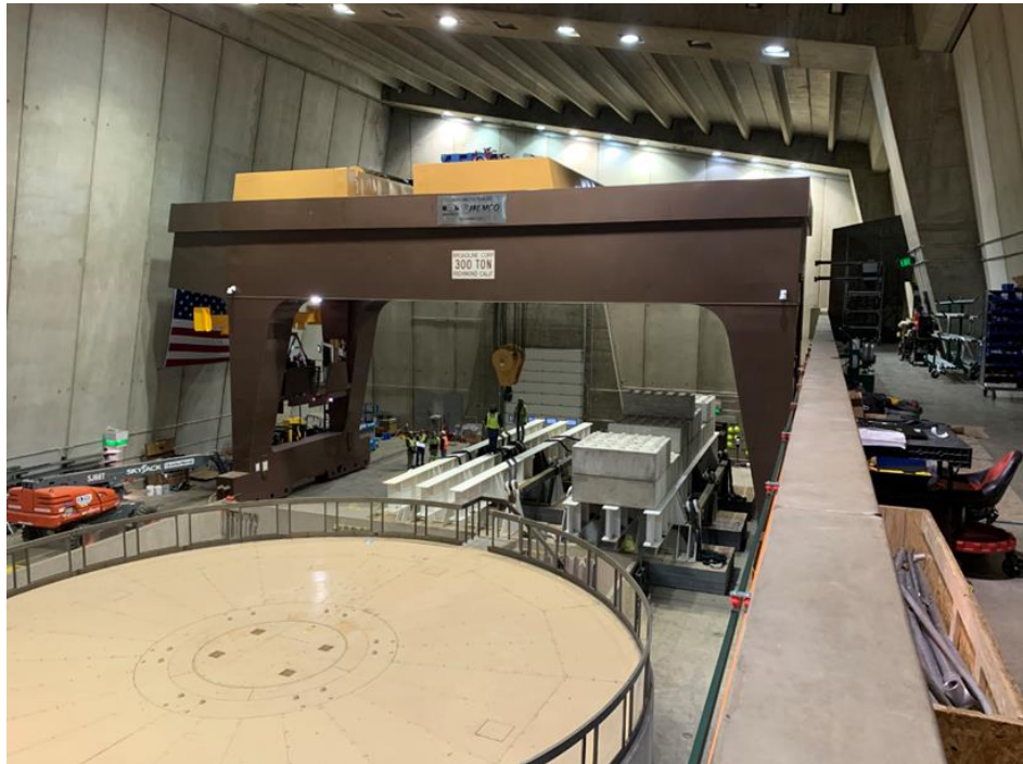
Figure 20-2. Powerhouse gantry crane
