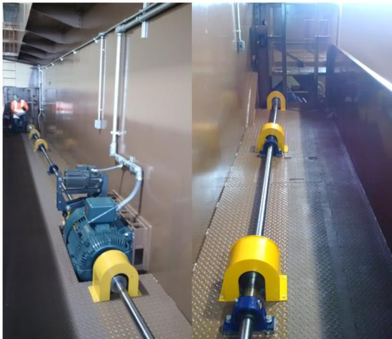
Figure 20–9. Powerhouse bridge crane with Crane Manufacturers Association of America A3 drive arrangement with all gear reduction located at each drive truck; gear reducer is partially visible in right image
