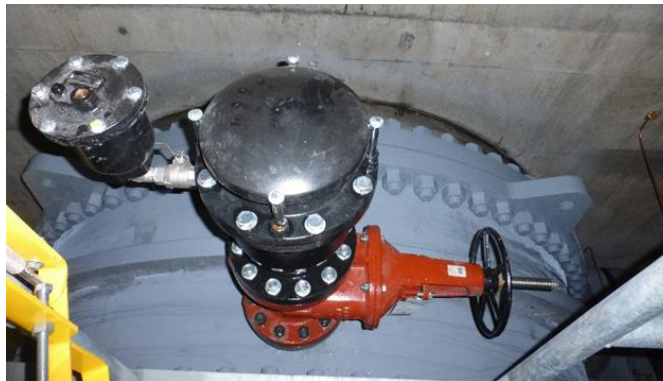
Figure 19–18. Air and vacuum breaker valve (black) with manual gate valve (red)
