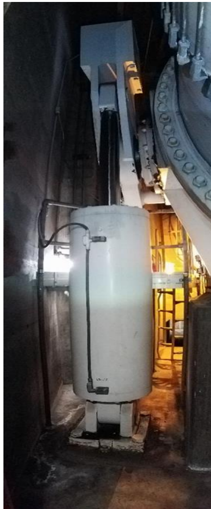
Figure 19–9. Vertical hydraulic valve operator for a horizontal butterfly valve with hammer-head closure weight (top)
