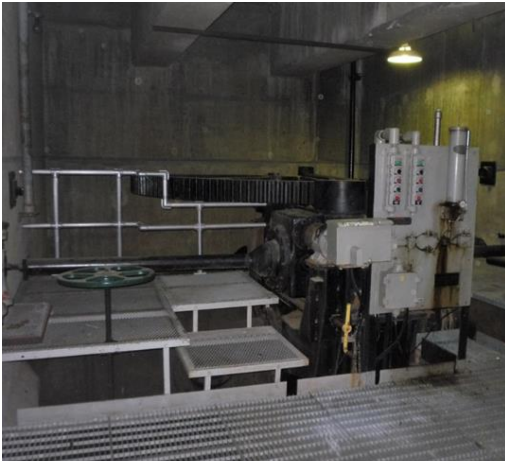
Figure 19–22. Platform access to valve operator and bypass valves that require no fall protection
