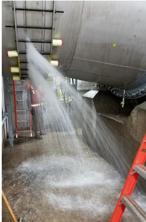
Figure 19–14. Leakage into valve operator room from scroll case extension slip-joint during initial setting of joint
