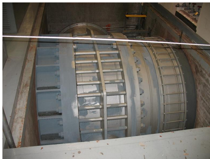
Figure 19–15. Flanged horizontal butterfly valve with bolted connection to penstock extension on left and scroll case extension on right
