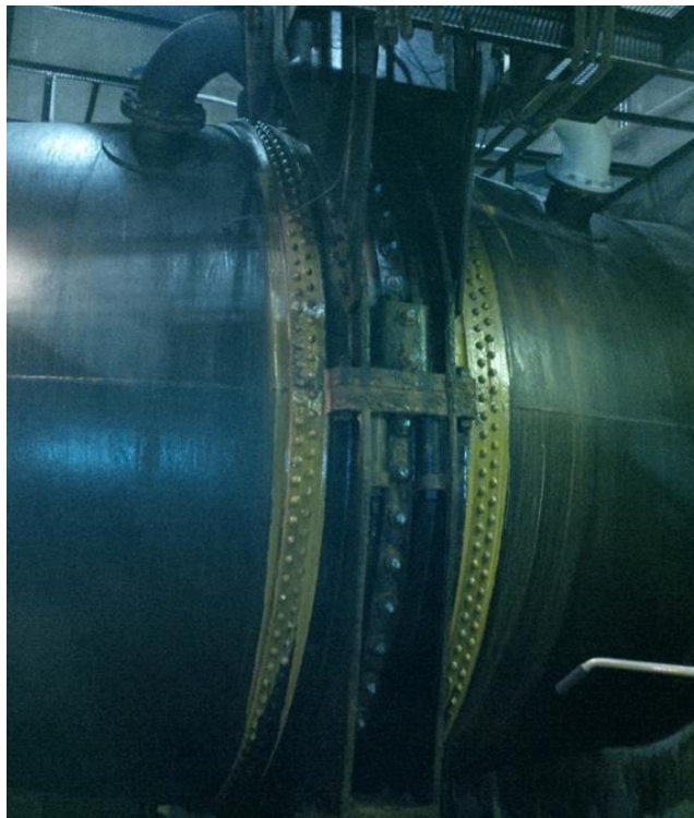
Figure 19–16. Vertical butterfly valve with riveted connection to both penstock extension and scroll case extension
