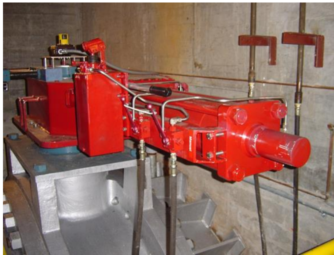
Figure 19–11. Horizontal hydraulic valve operator for a vertical butterfly valve
