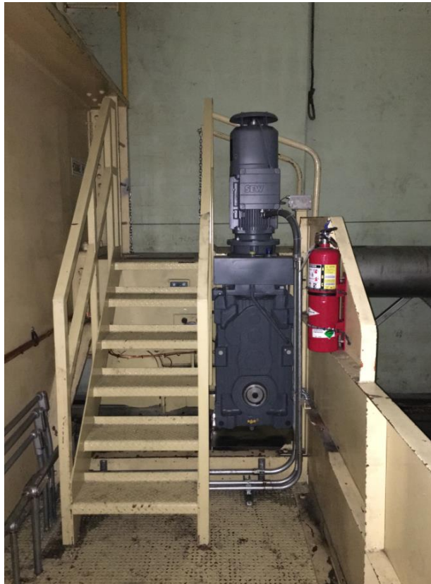
Figure 20–11. Powerhouse bridge crane with Crane Manufacturers Association of America A4 Type 2 drive arrangement
