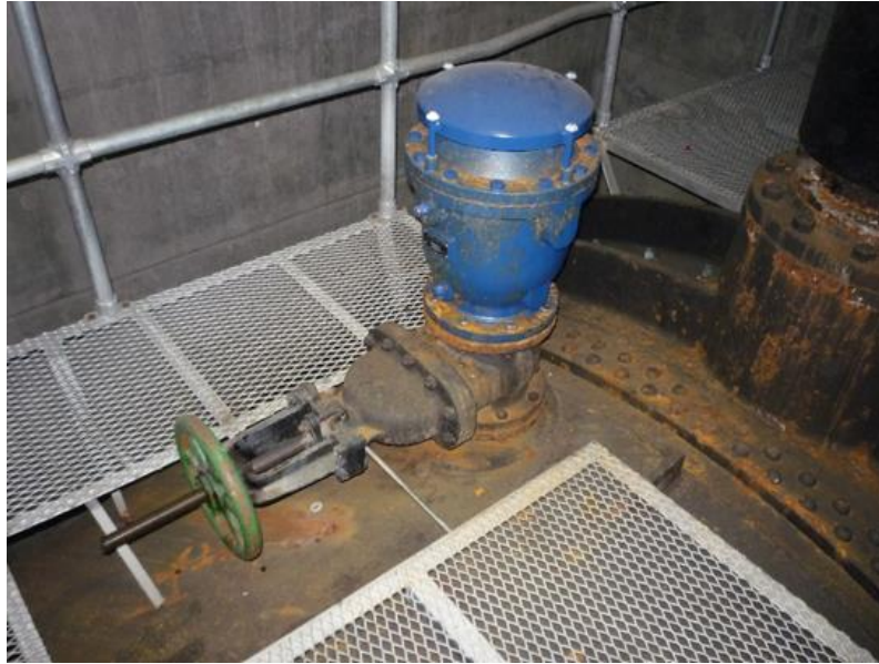
Figure 19–23. Platform access around air and vacuum breaker valve assembly requiring no fall protection
